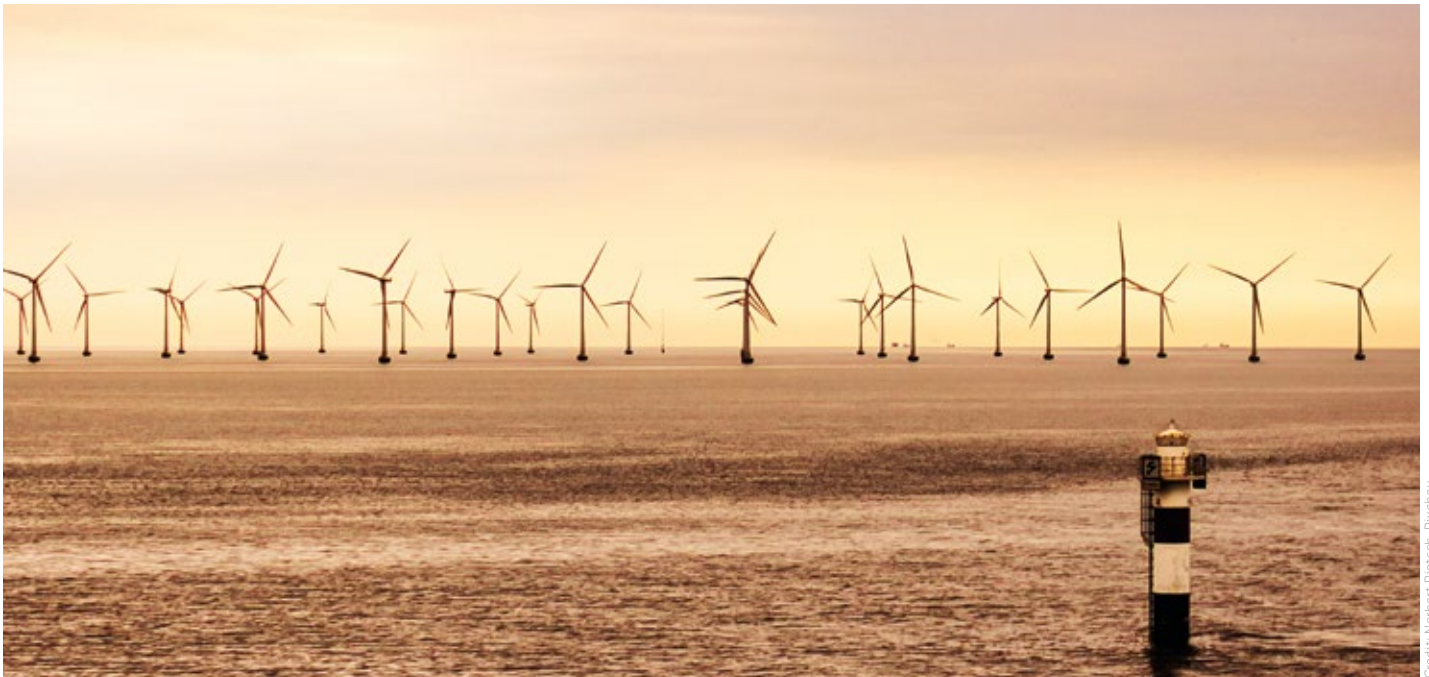
Wind turbines at sea.
