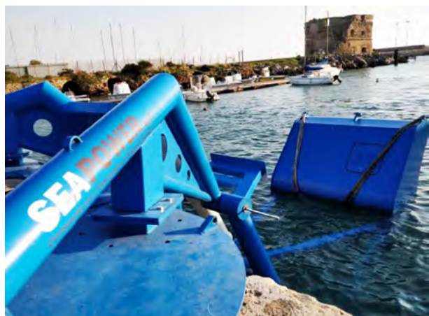
Pivot installation in Civitavecchia
