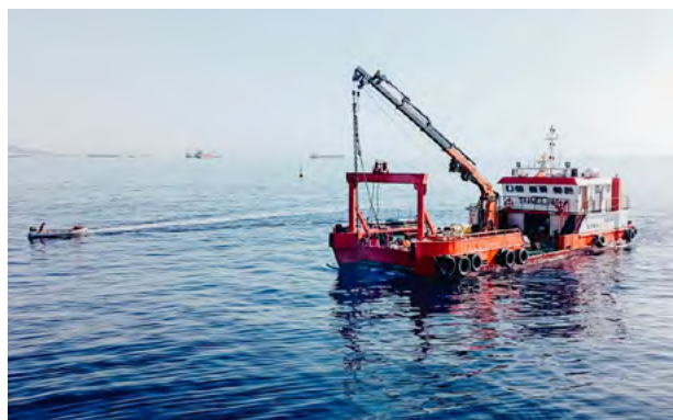
Installation of Wavepiston
