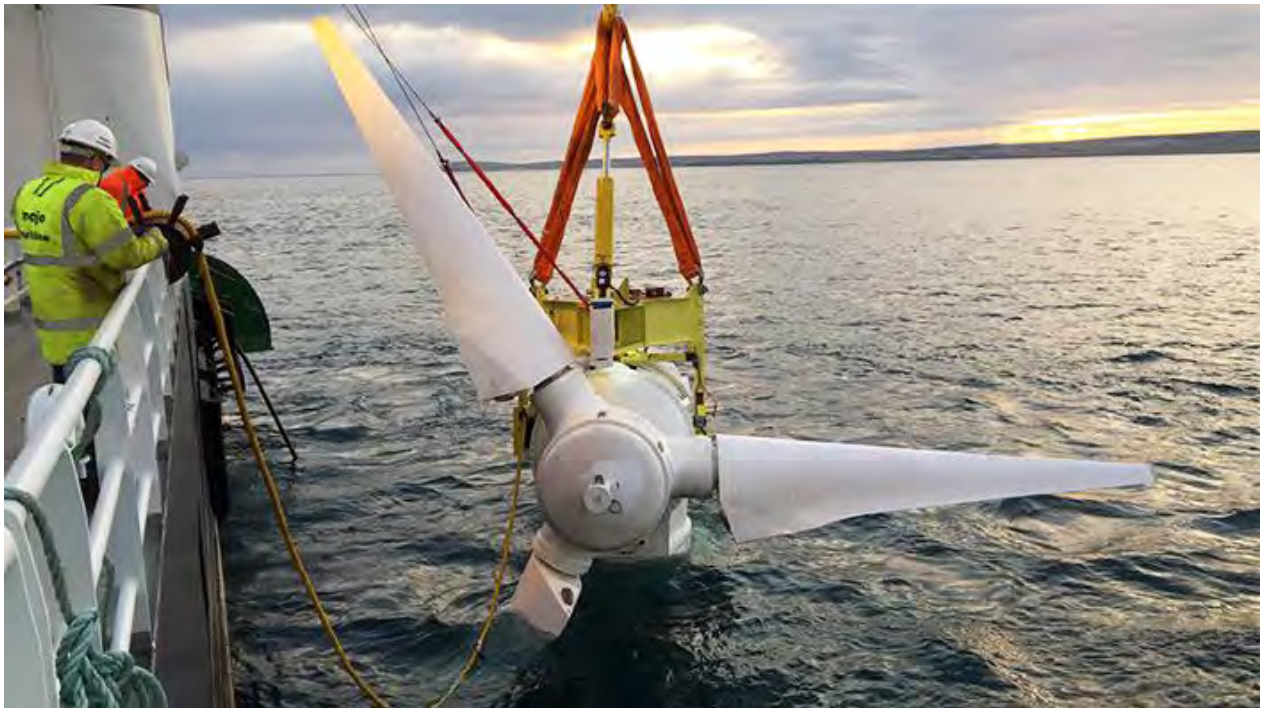
A MeyGen turbine is lowered beneath the waves (Credit: SAE Renewables)
