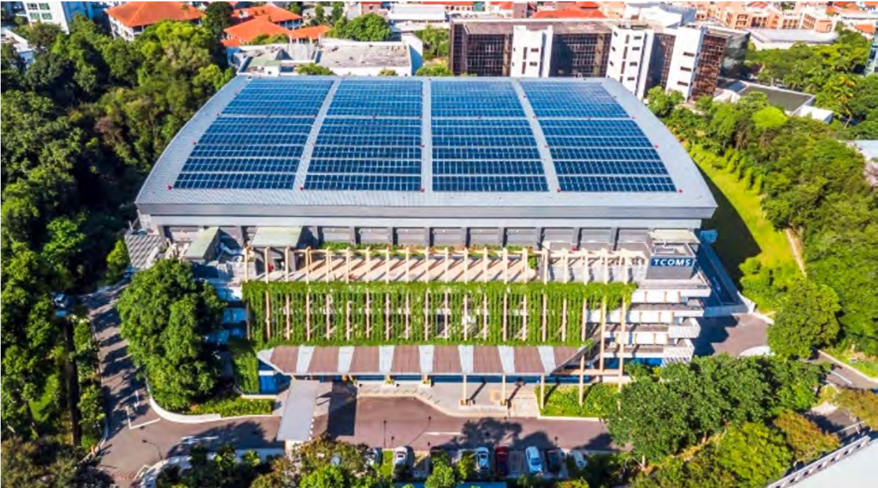
TCOMS – Ocean basin Facility
