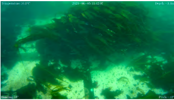
Anchor block inspection (June 2023)
